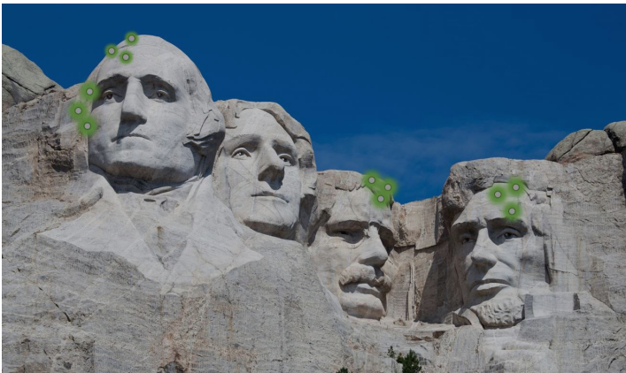
Luna sensors monitor four separate regions on the monument for strain and temperature
