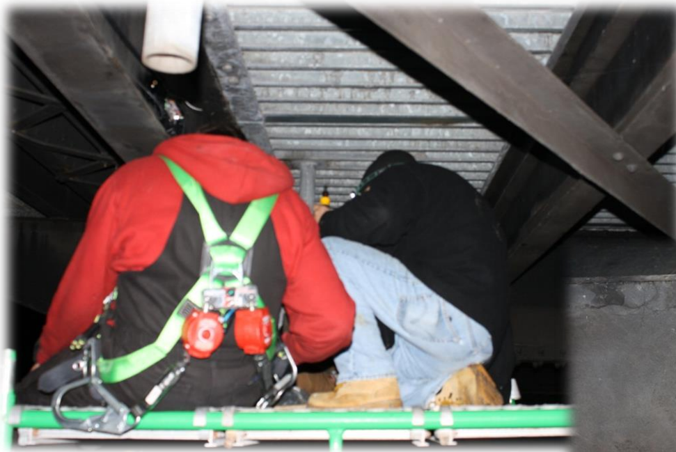
3D Accelerometer being installed on the swing span
